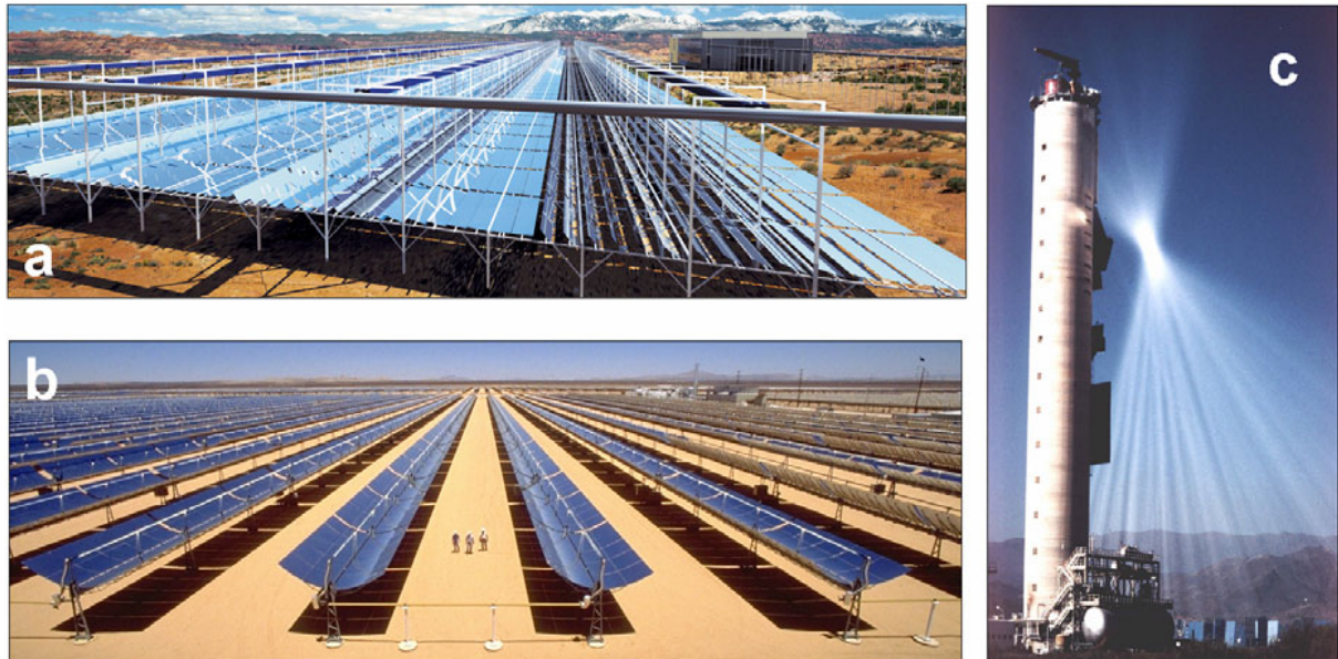
Fig. 1. Concentrating solar collector systems with (a) Fresnel concentrators (picture: computer simulation); (b) parabolic trough concentrators; and (c) the solar tower concept with surrounding heliostat field.
